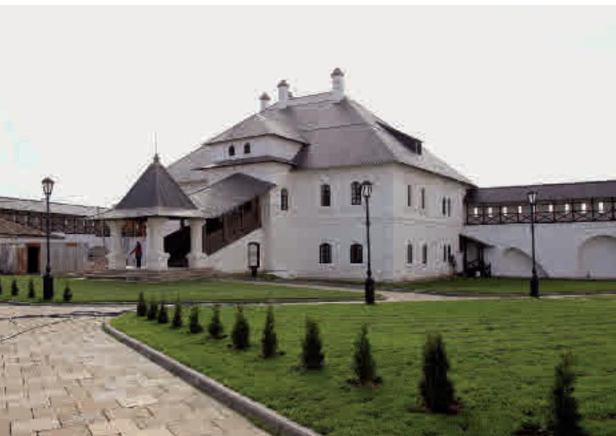
the arrangement of the planked roof, the arrangement of the chimneys, assembly of the window and door openings, interior finishing, arrangement of the wooden and white-stone floors, provision of furniture and kitchen equipment, arrangement of the discreet perimeter walks, development of the adjacent area. The building was fully provided with utilities.
