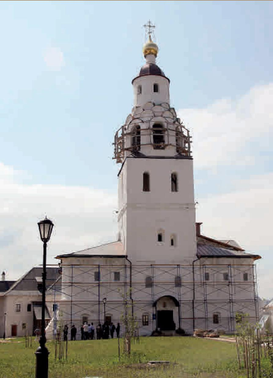
the bell-tower, arrangement of the drainage system, partial cleaning of the vaults, injecting of cracks in vaults and walls, restoration of the window assemblies, restoration of the cross, restoration of the facades, arrangement of the window and door assemblies, restoration of the stairs, restoration of the top with a drum in the northern side-altar of the temple, arrangement of the discreet perimeter walks.
