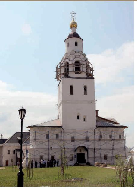
the bell-tower, arrangement of the drainage system, partial cleaning of the vaults, injecting of cracks in vaults and walls, restoration of the window assemblies, restoration of the cross, restoration of the facades, arrangement of the window and door assemblies, restoration of the stairs, restoration of the top with a drum in the northern side-altar of the temple, arrangement of the discreet perimeter walks.
